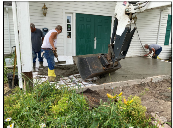
Men Pouring Concrete in front of the Myra Museum Entryway
